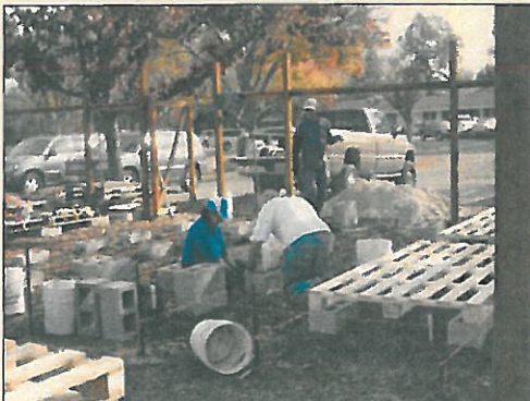
Images from left to right: 1) Aligning and leveling the last row of blocks. On the right, a finished row with pallets in place. 2) Building the plant frames. It took one to staple, two to keep the hardware cloth aligned and taut, and one to steady the frame. 3) Unloading plants from Don's big truck at the nursery.
